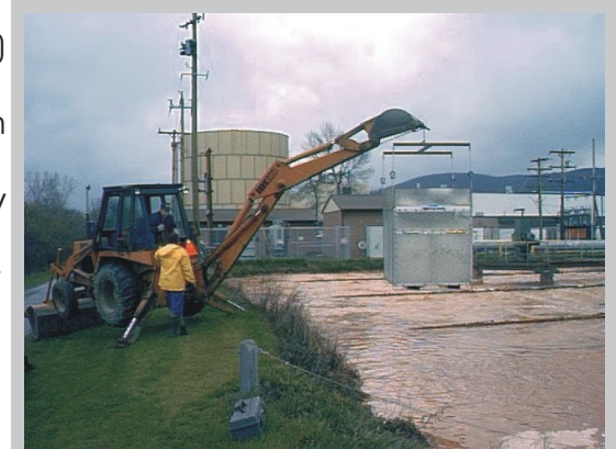
Bio 2 Bloc system being installed with a back-hoe.
