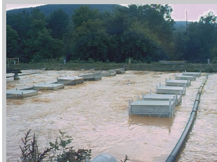
After Bio 2 Bloc installation
