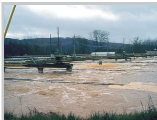
Before Bio 2 Bloc installation
