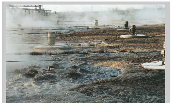
O 2 ctopus system efficiently diffuses air 8 ft. below the surface.
